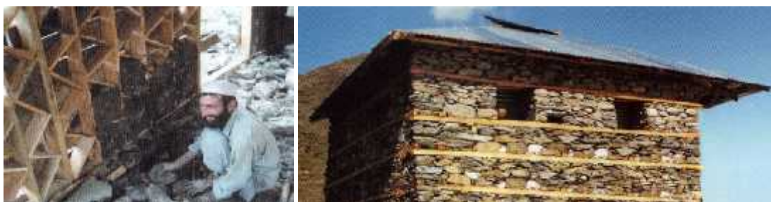
Figure 4: (Left) Construction process of KotDhijji method using wooden diagonal bracings. (Right) BahitterTarz-e-Tameer with horizontal wooden elements
